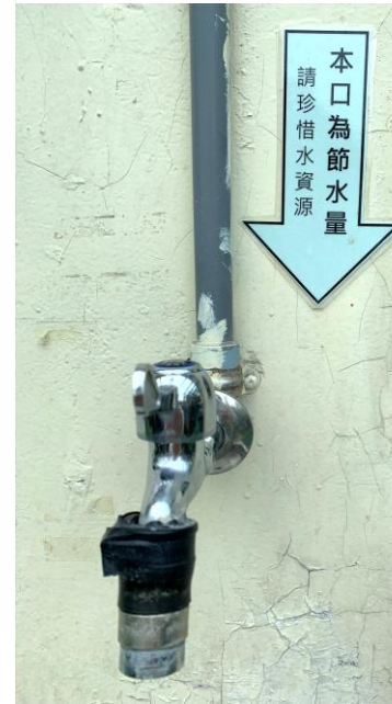
Faucet water-saving devices and slogans installed.
