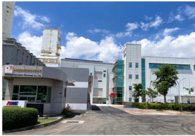
Taichung Photonics - FAB Expansion Project
