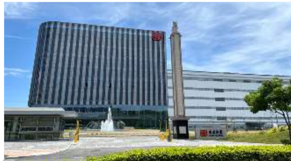
Kaohsiung Campus Construction Project for Garuda Technology
