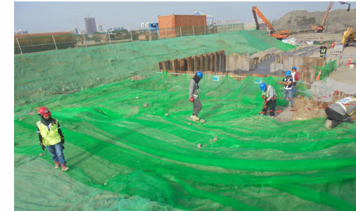
Falsework - Green Grid
