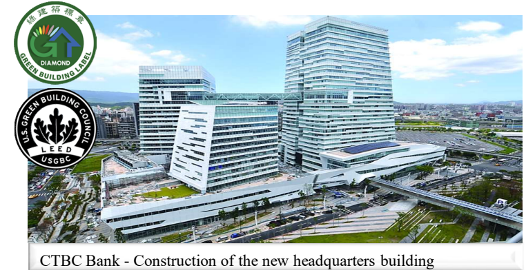
CTBC Bank - Construction of the new headquarters building
