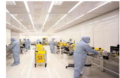
Energy-saving Lighting Equipment
